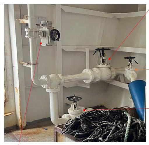
Overboard discharge manually operated valve, **kept open**
